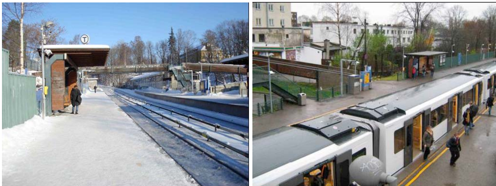
Figure 25 : Overview of the station with its two platforms and the pedestrian bridge.
